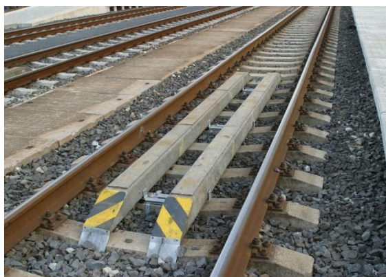
Left picture: Track-side part of the ATO - magnetic information point (photo: www.fscr.cz )
