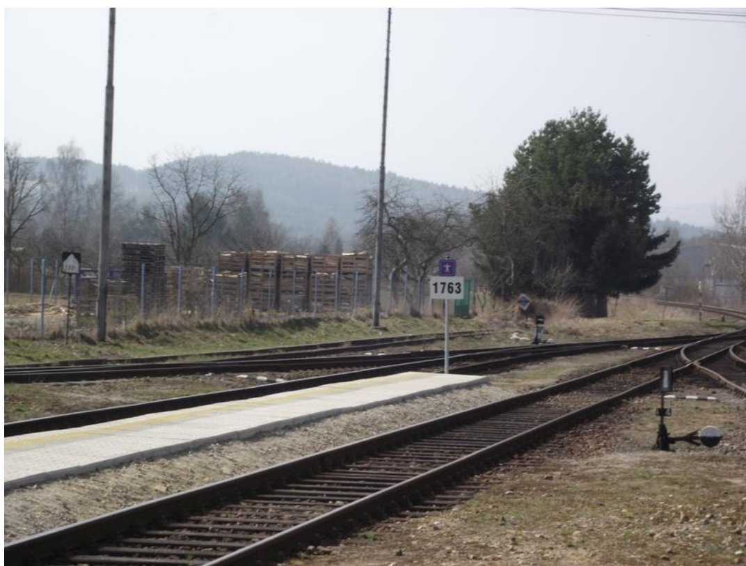
Picture: The trapezoid sign board in the front is the border of operating post D3 Havlovice located near to branch Pasečnice, where the regional line to Planá u Mariánských Lázní depart from the main line from Pilsen – Domažlice to Česká Kubice – Furth im Wald (Bavaria) (photo: Tomáš Paška, www.strojvedouciplzen.cz )
