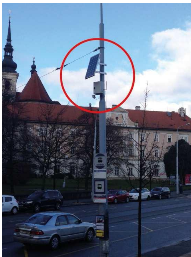
Master - CM 1212 (60 W PV panel, 33Ah aku)
